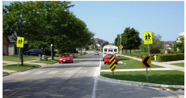
An appropriate motor vehicle **curb radius** is achieved through a curb extension, which also shortens the crossing distance and increases space for green infrastructure.
