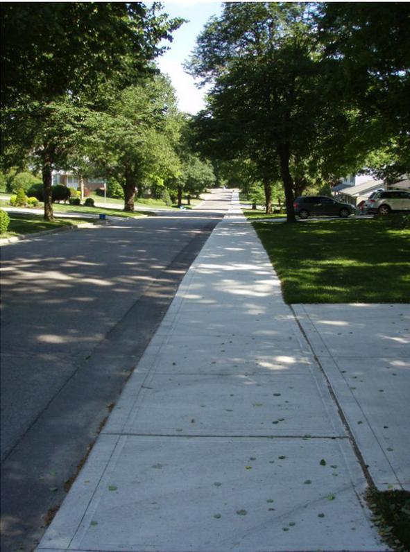
While a 1.0 m minimum offset from the curb is preferred, **sidewalks that abut the curb** are appropriate in constrained areas and retrofit applications where the 1.0 m offset is infeasible.
