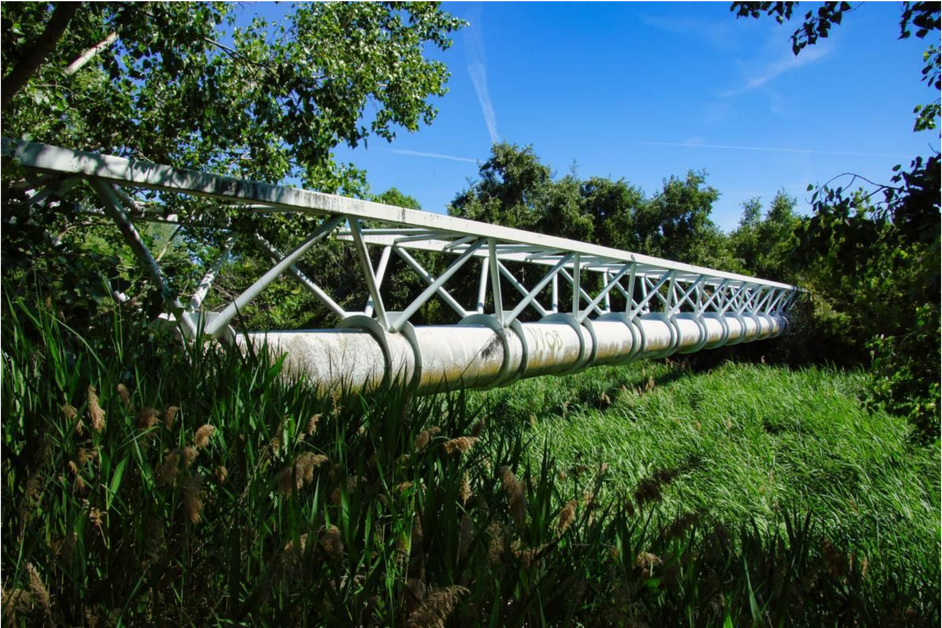
Figure 4: Gravity Sewer Strapped to Structure (Example) Source: structurae.net
